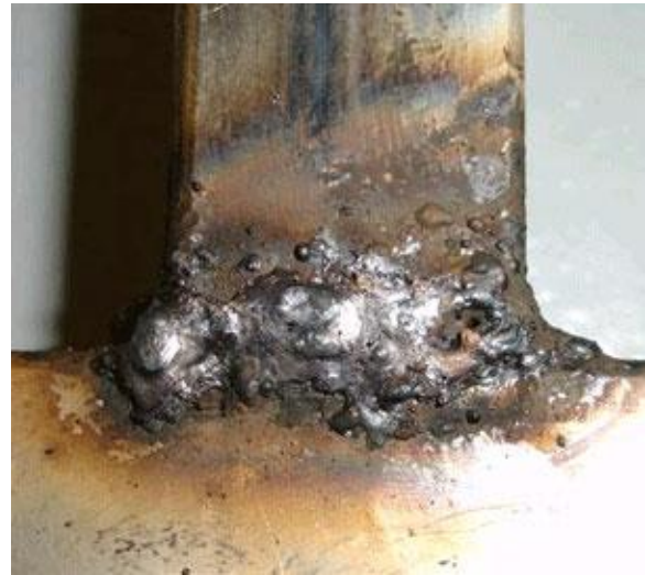
Figure 409.1.3 (3) Poor Quality Weld Image
